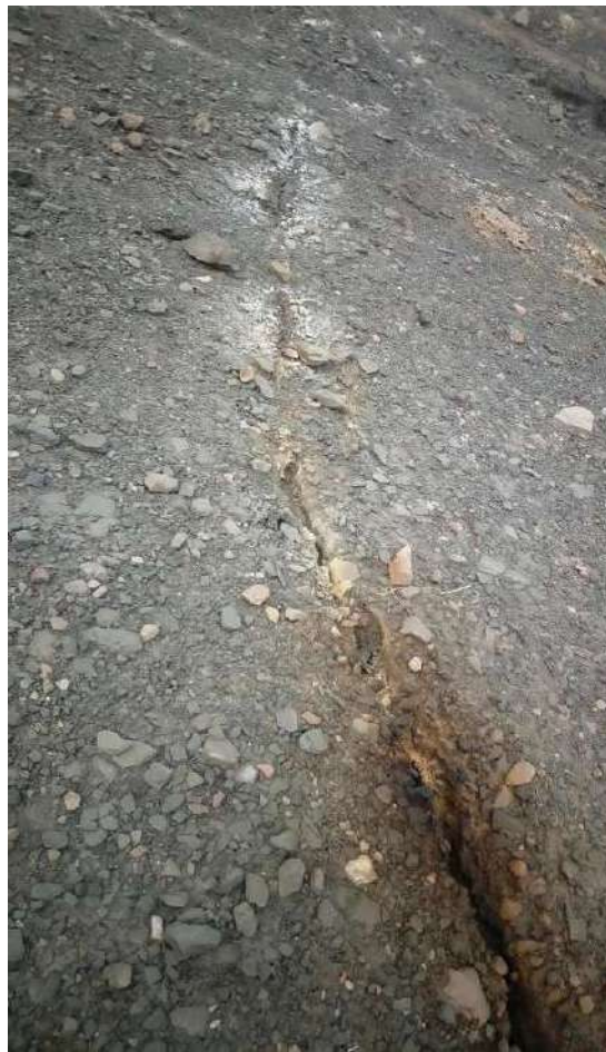
Figure 20: Fume cracks in the Bhulanbarari area.
